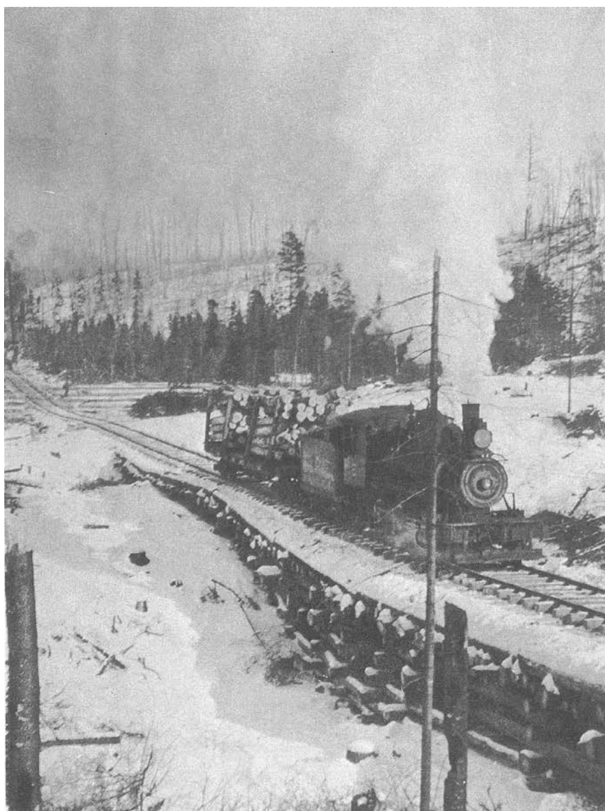
Blasting up a steep grade, a Duluth and Northeastern engine moves one flat of logs at a time, as steam jammer at the end of the spur loads another car. Unballasted track and fill work in the deep cut where typical on these temporary spurs.
