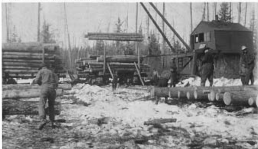
Loading logs with a steam jammer (above) in Brooks-Scanlon Camp No. 17 north of Duluth about 1907. Below is a nice, average, four-horse load of logs near Mizpah in 1917.
